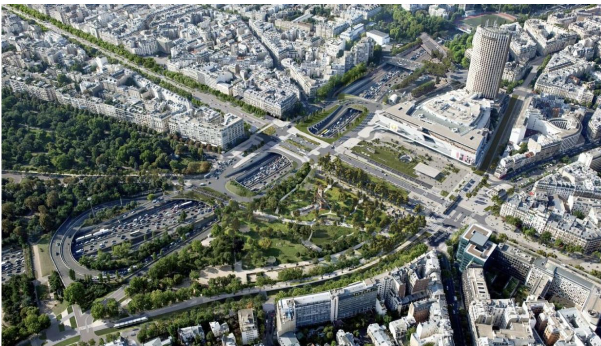
An overview of the remodelling of Porte Maillot, showing how gardens and walkways will partly cover the Boulevard Périphérique. Photo: ©PCA-Stream
